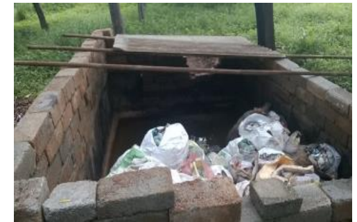
Waste Storage Tank
